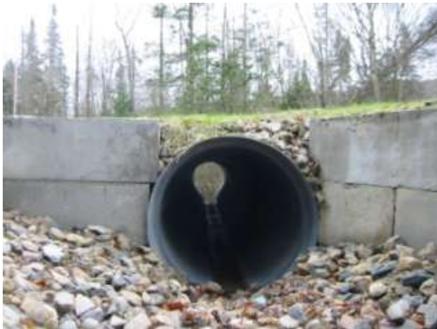
New culvert on Lincoln Road north of the intersection with Pearl Lee Road, a 2012 VTrans Structures Grant project
