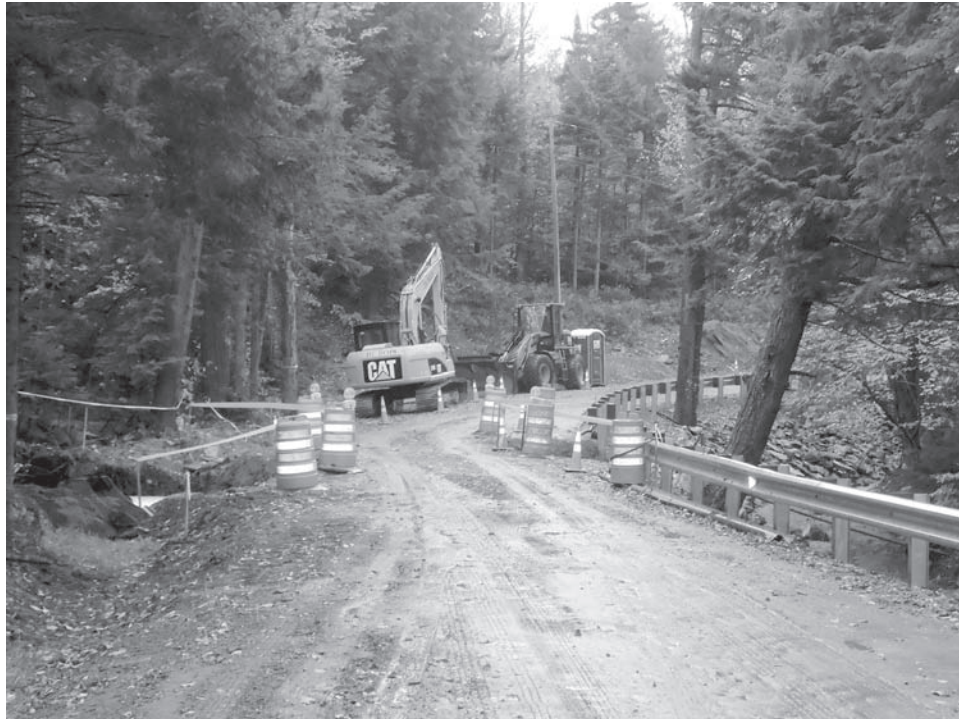
West Hill Culvert October 2012
